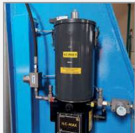
Automatic centralized lubrication system with timer and monitored distributors
